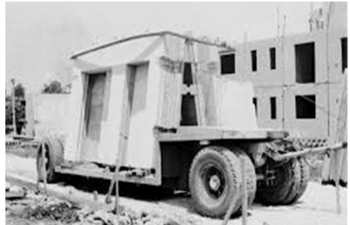
Fig. 7. Vehicles with trailers suitable for transporting precast panels to the construction site © AQTN
