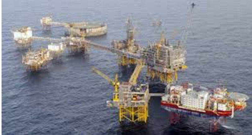
Crude oil production platform. Source-Electrical engineering portal.com
