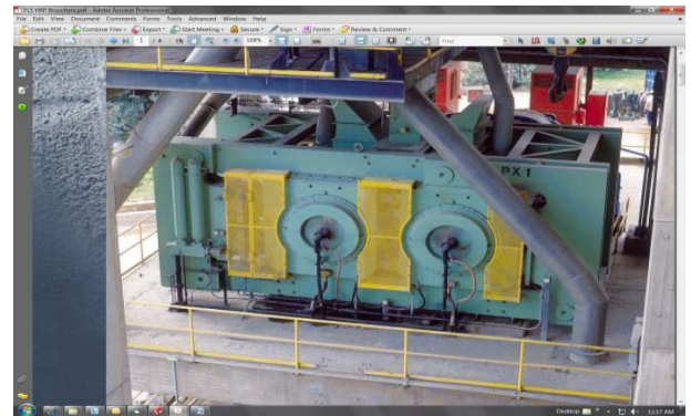
Fig.2 Hydraulic Roller Press at site
