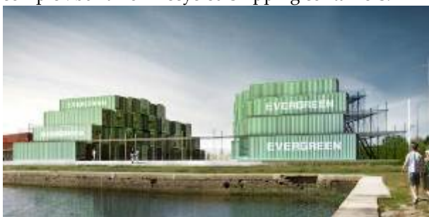
Figure 35: 'Crou' student housing made from 100 recycled shipping containers
