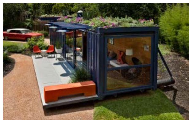
Figure 14: the guest house green roof .
