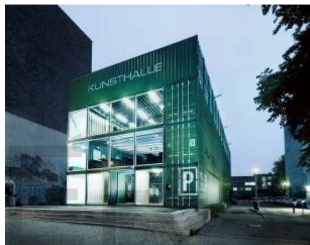
Figure 31: creating a transparent elevation by removing the doors and replacing them with glass panels.
