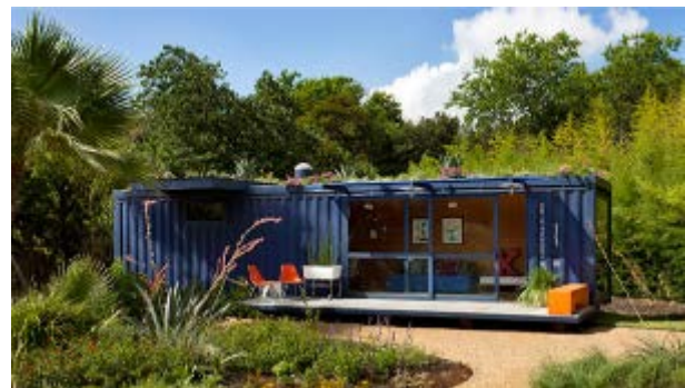
Figure 12: the integration of the guest house with the surrounding environment.
