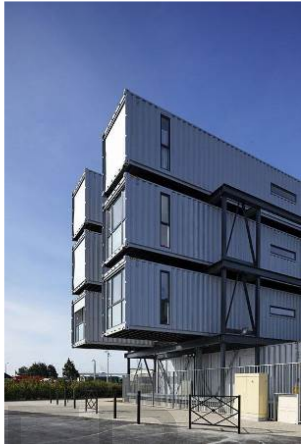
Figure 27: a steel skeleton was constructed to host the containers.
