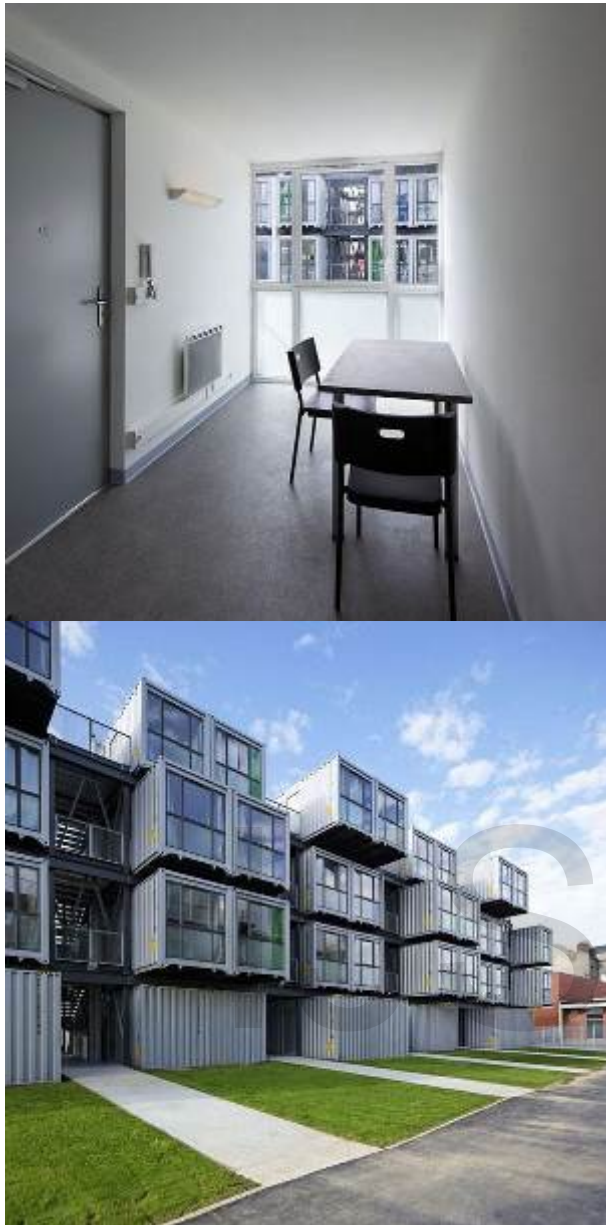
Figure 27: a steel skeleton was constructed to host the containers.
