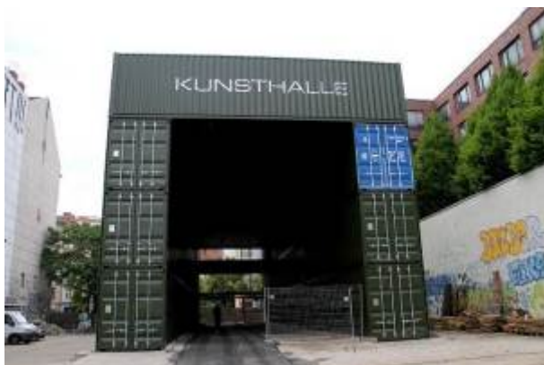
Figure 29: vertical stacking of containers lead to a reasonable height that is suitable for art works display.
