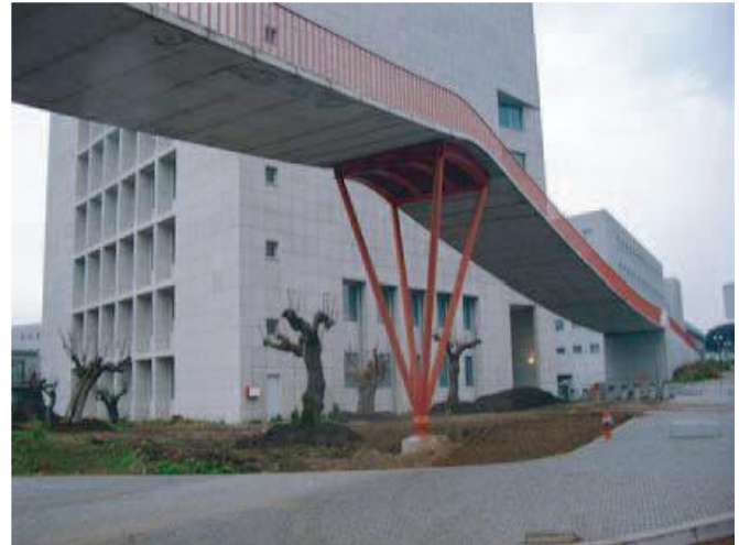
Figure1: Typical Stress Ribbon Bridge
