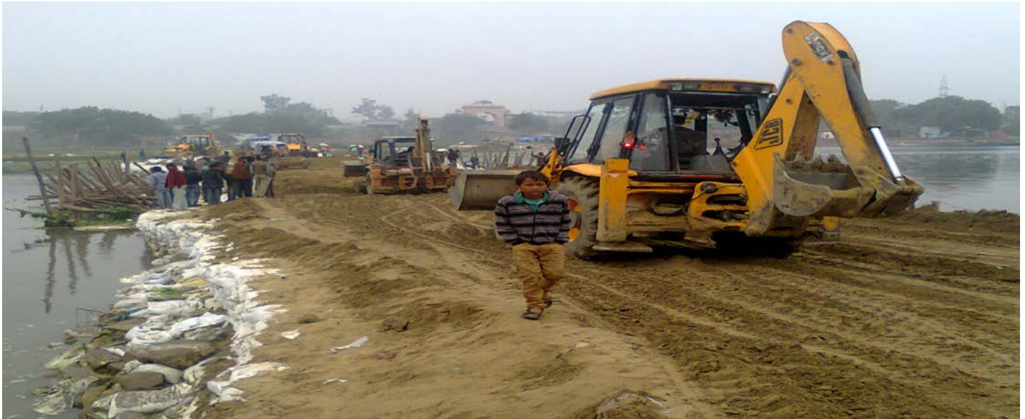
Photograph :- Execution of Dam As Designed Above.
