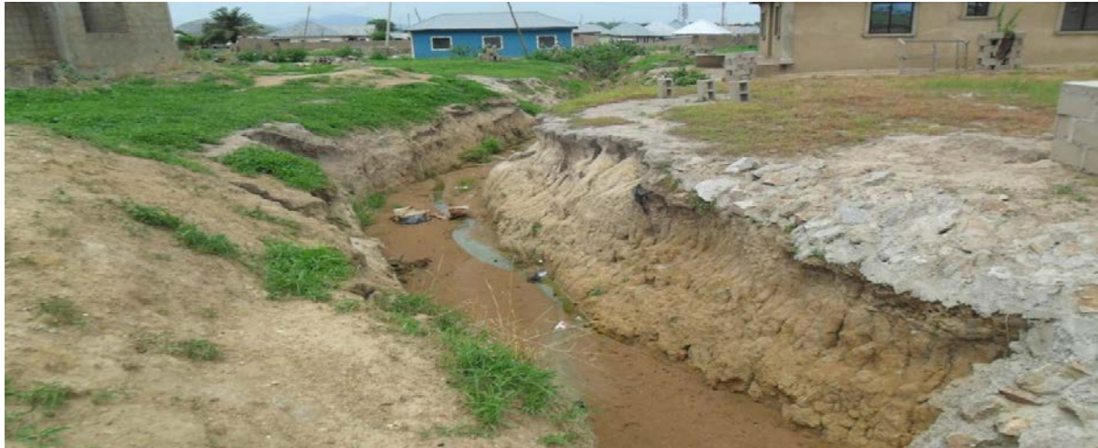
PLATE 3: Gully erosion in Abuja phase II, Jalingo (Source: Field Survey, 2012)
