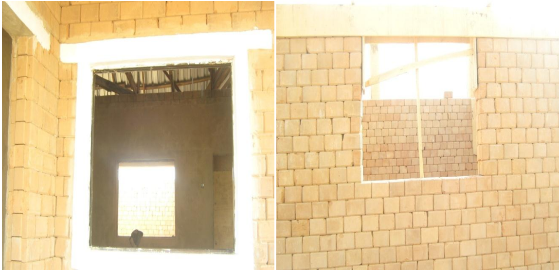
Figure 2 250 blocks not completed after 120 days expired
